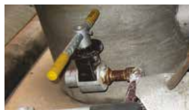
Instrument Sensor Isolation Valve
