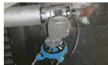
Water Wall Drain Valve
