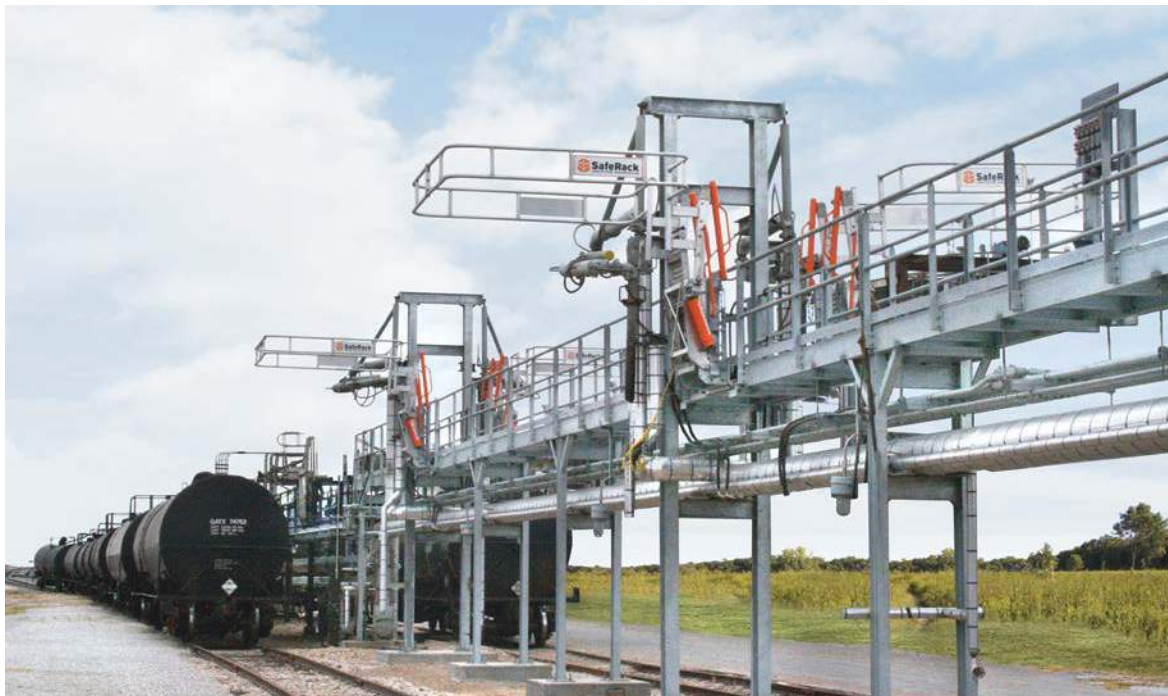
Loading arms with supports integrated into SafeRack platform system. /
