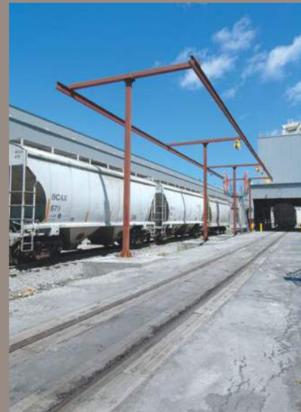
Primed steel trolley beam system with SafeRack for access. /
