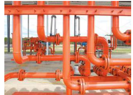
Ethanol & biodiesel combination blending skid. /
