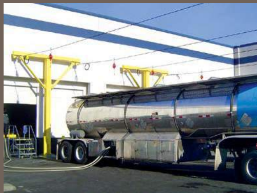
Permacable fall protection system for tank trucks. /
