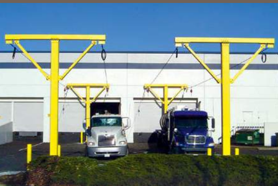
Four-bay Permacable lifeline system. /
